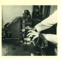
9. Turn the machine to 200° and place the mould blade slide in the backward position.
